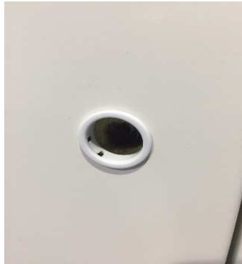
Metal Door Cap removed, Collar exposed
