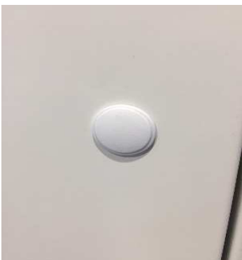
Metal Door Cap & Collar installed
