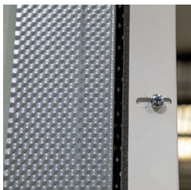
Ensure the foam gasket has been compressed by the frame channel to ensure a good seal with the substructure.
