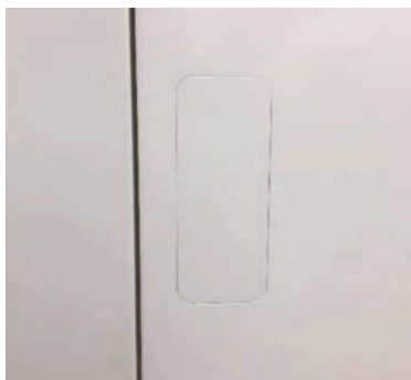
Cover installed flush
