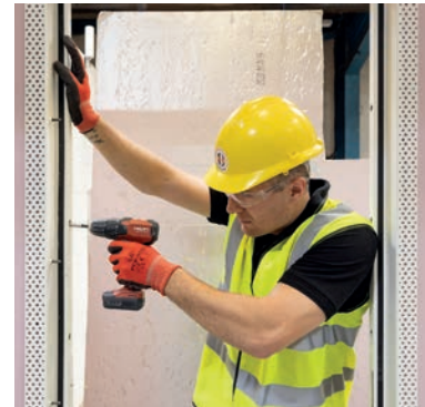
Secure the self-adjusting frame to the stud work through the side fixings using suitable substrate screws.
