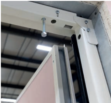
Insert the jacking screws top and bottom if they are not already fitted into the frame.
