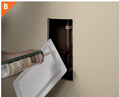
Silicone adhesive is applied to the inside edge of the picture frame
