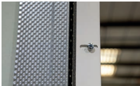
Frame adjusts to fit each structural opening, no plastic packers required
